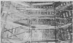
New easy to build and flexible to use scaffolds all around inside the 80-ft. high furnace assure stability and safety.
